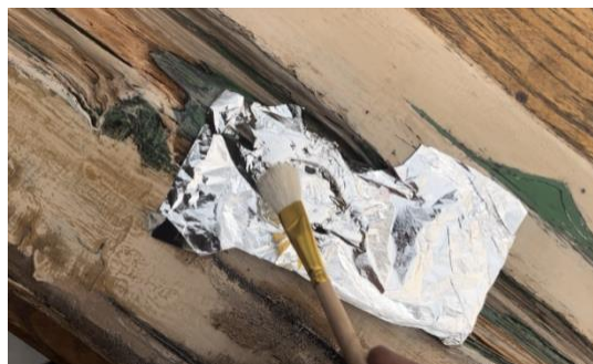
Figure 8. Lacquer and apply aluminum foil.
